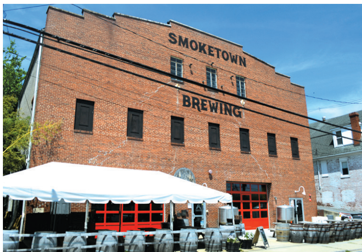
Smoketown Brewing Station at 223 W. Potomac Street
