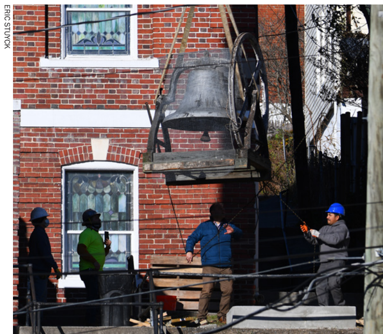
Workmen lower the First Baptist Church bell to the ground.
